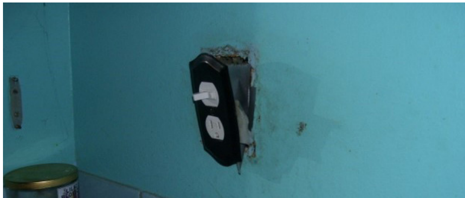
An electrical outlet protruding from the wall and covered with duct tape. Source: U.S. Department of Health and Human Services' Office of the Inspector General.
