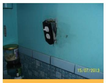
An electrical outlet protruding from the wall and covered with duct tape.
