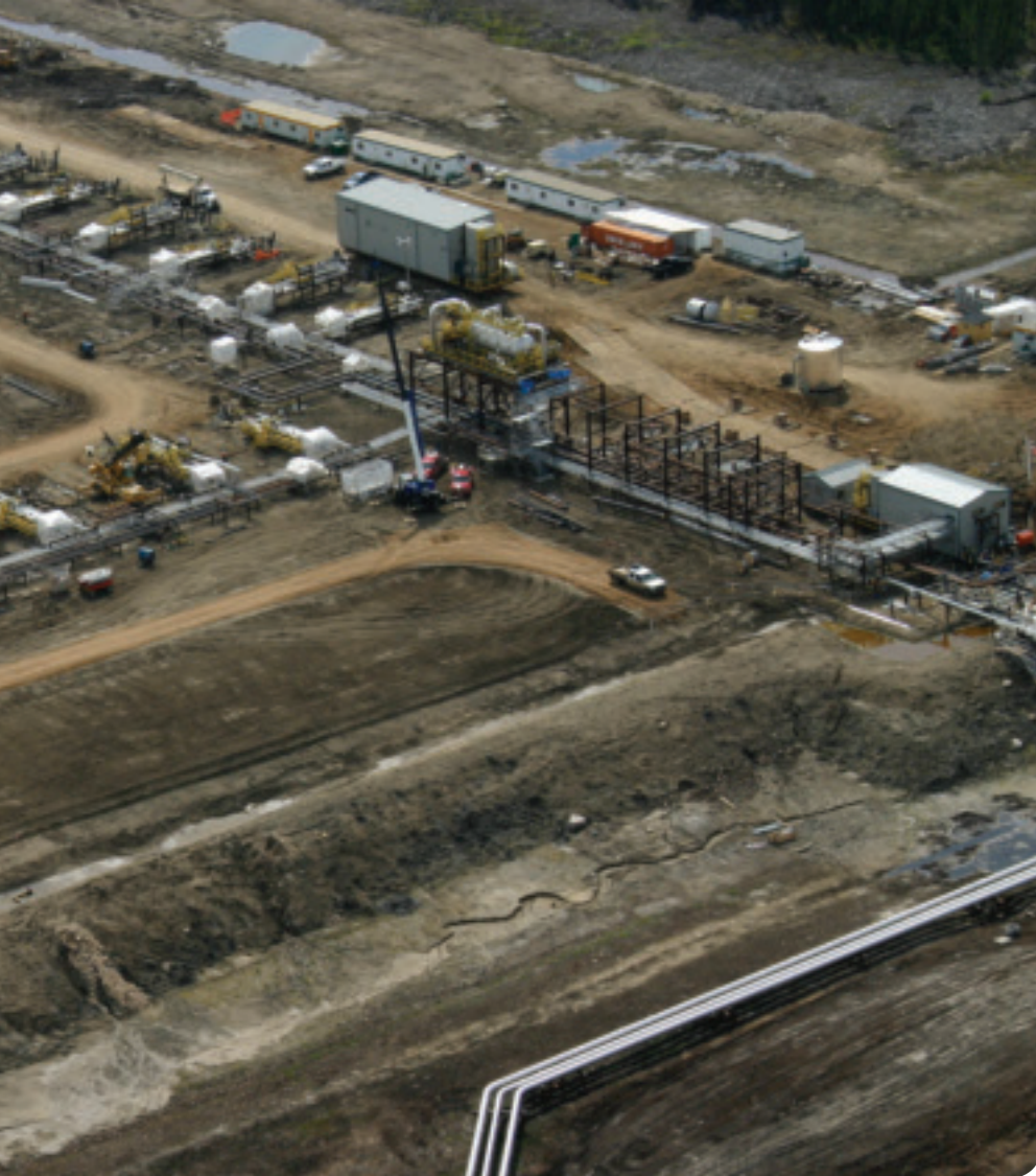
Pipelines transporting steam and bitumen for oil sands production.
