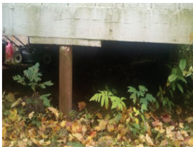
A crawl space beneath a provider's home that was accessible to children.
