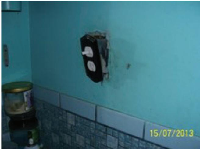
An electrical outlet protruding from the wall and covered with duct tape.
