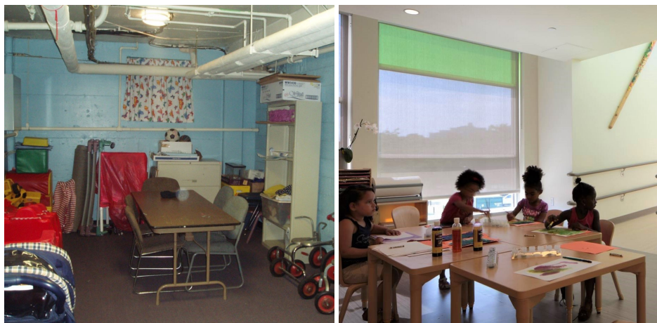
Nurtury Learning Lab in Boston, Massachusetts, was located in a basement of a public housing development for years before moving to their new location. After its renovation, includes natural light and child-sized furniture. Photos provided by Children’s Investment Fund.
